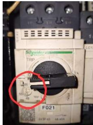
Figure 6. Setting overload
